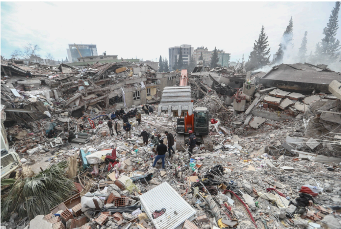
Damaged buildings in Kahramanmaraş after 7.8 magnitude earthquake in Türkiye (2023) by Əziz Kərimov (VOA)
